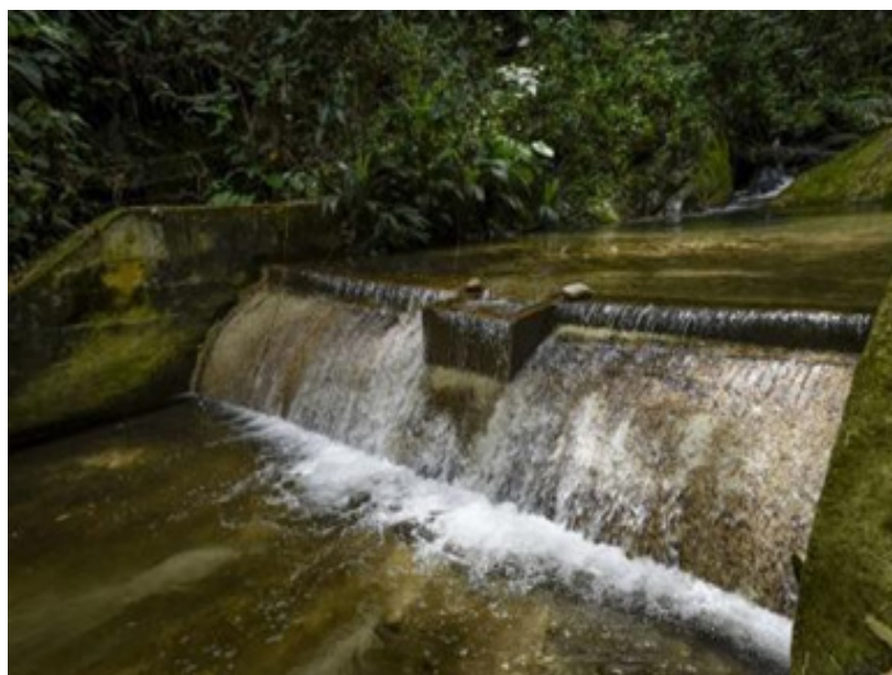
Figure 2. Aguablanca Creek Catchment Structure El Topacio Plant
