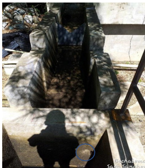
Figure 17. Water inlet to the first chamber of the flocculator
