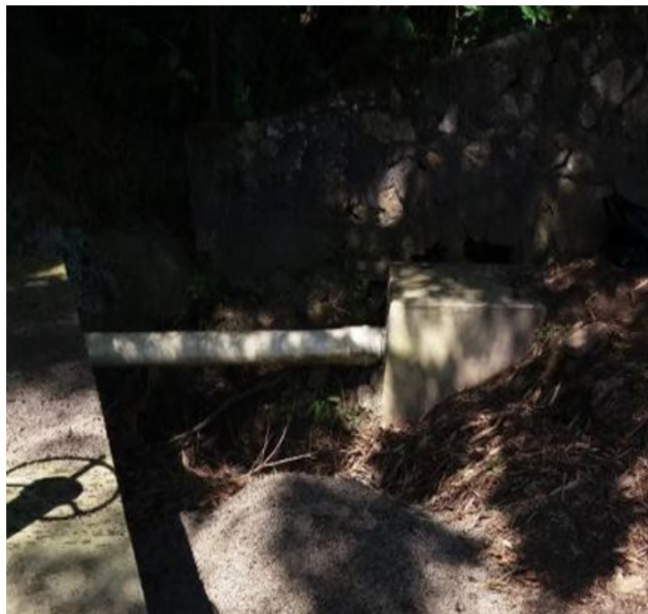
Figure 4. Entrance channel to the desander
