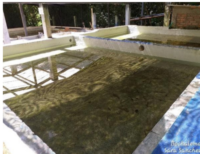
Figure 11. Upflow Fast Filter
