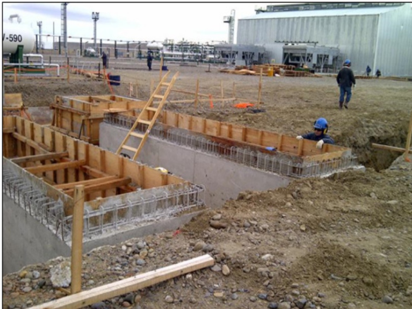
Figure 9. Chamber formwork
