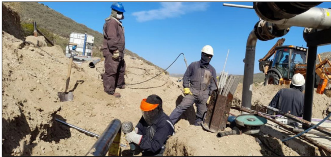
Figure 5. Operator is planing pipe 4 with 750/115 mm angle grinder
