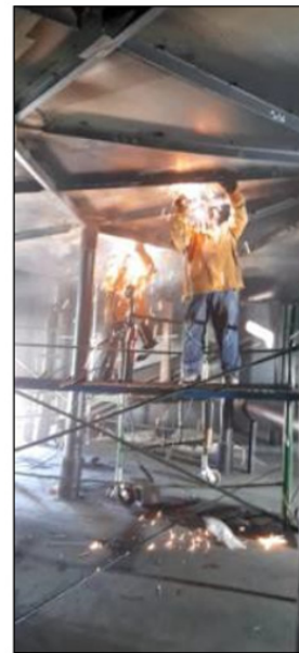
Figure 6. 4-5 Confined space welding with scaffolding on cutting tank, south floor
