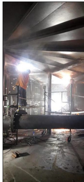
Figure 6. 4-5 Confined space welding with scaffolding on cutting tank, south floor
