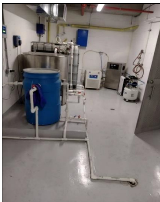
Figure 17. Photograph of the ozonation process installed at Imbanaco Medical Center
