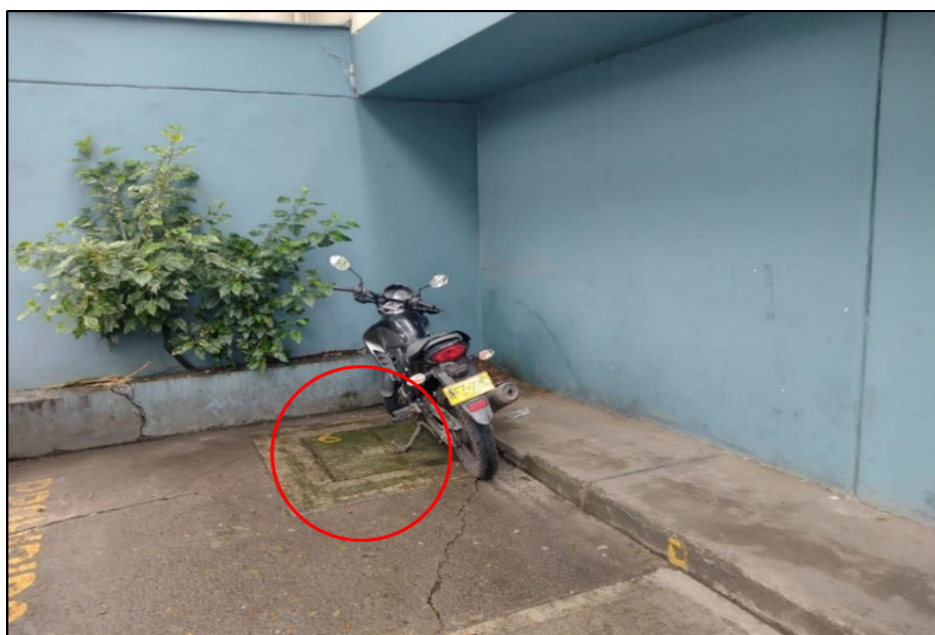
Figure 10. Tower A monitoring point 5
