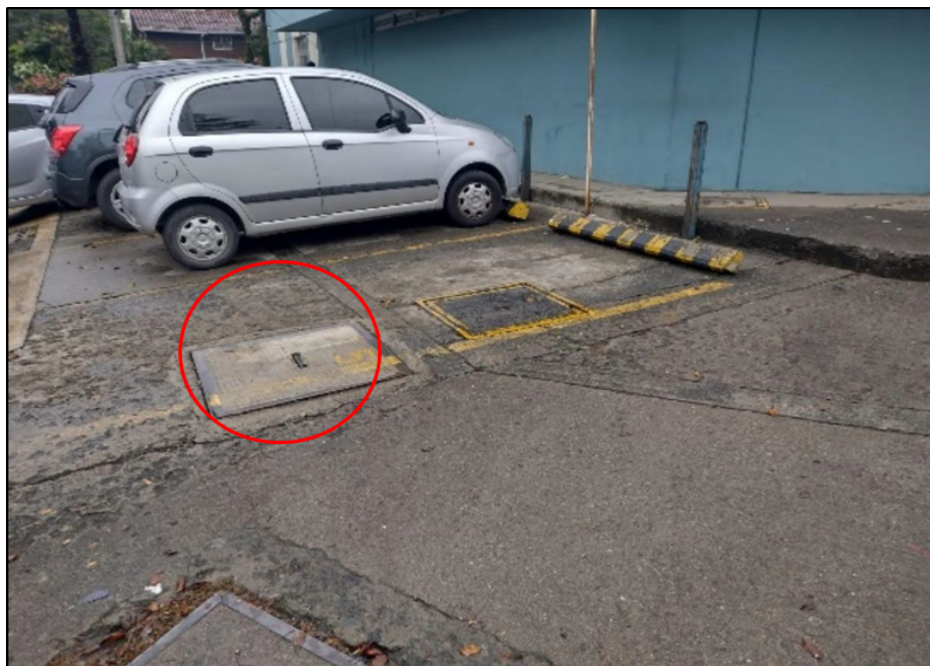
Figure 9. Tower A monitoring point 4
